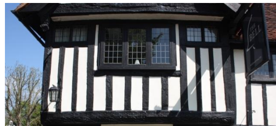
Fig. 2 Exposed timber framing on The Bell
