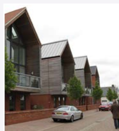
Roof overhangs providing protection to glazed facade
