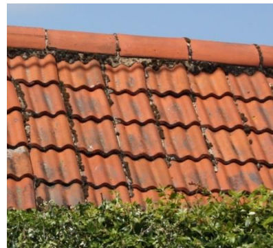
Fig. 11 Single-lap clay pantiles
