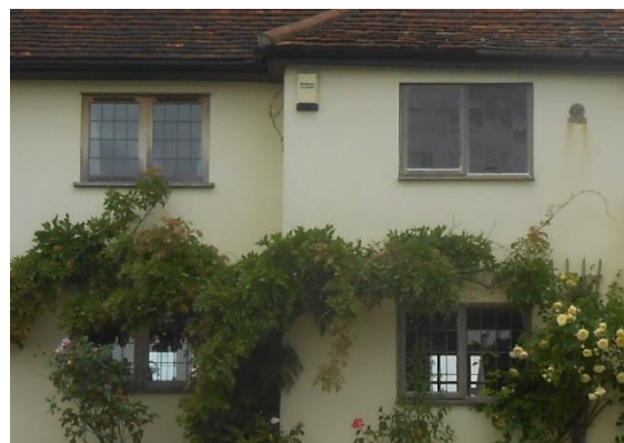
Fig. 17 Lead-glazed windows in unpainted oak frames
