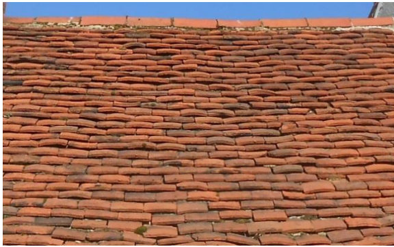
Fig. 10 Double-cambered clay plain tiles
