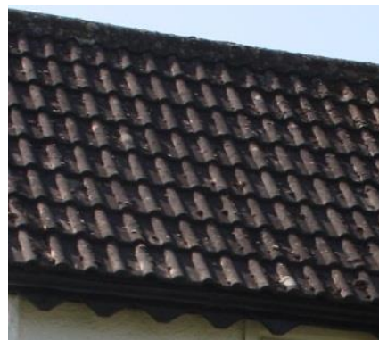
Fig. 13 20 th -century concrete tiles
