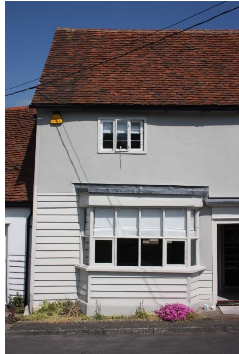
Fig. 1 Render above weatherboarding on Wingtons
